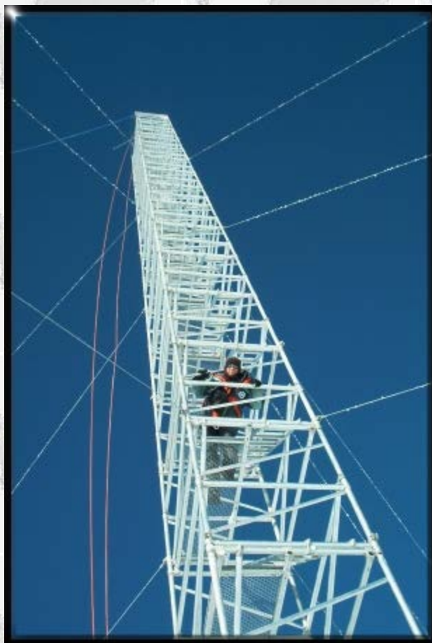
The 33 meter tower, a platform for instruments that measure snow surface reflectance. Photo by Richard Brandt.
